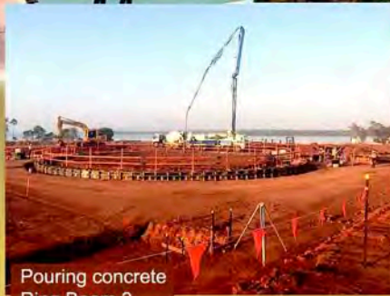
Building the Tank Farm walls
